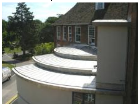
New Reception Roof
